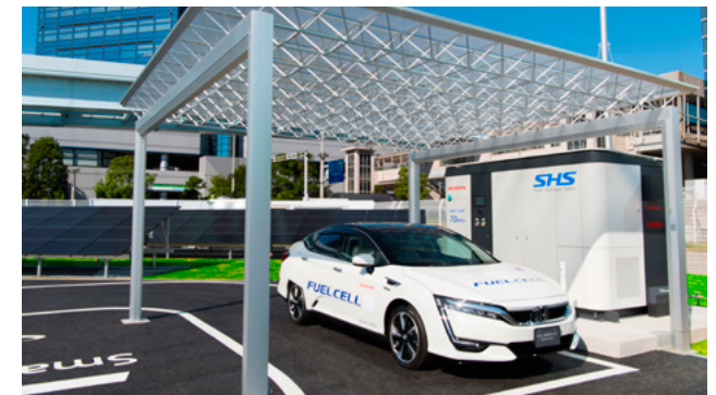
A Smart Hydrogen Station (SHS) producing 70MPa hydrogen
